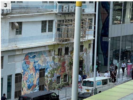
Graffiti on facade of Sing Tek Factory Building on Wong Chuk Hang Rd, Oct. 8, 2025
